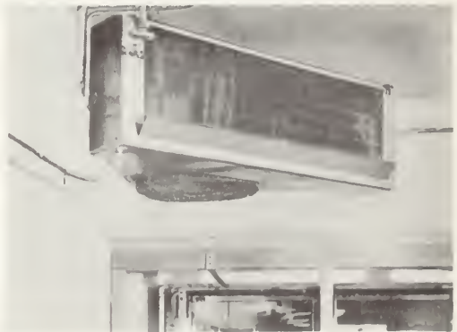
19-23. A blower coil designed for mounting in the corner of a refrigerator. Note the small amount of space required. The air enters at the bottom, is cooled and exits at the front. The unit requires a liquid line, a suction line, an electrical line, and a drain pipe. (Refrigeration Engineering, Inc.)
